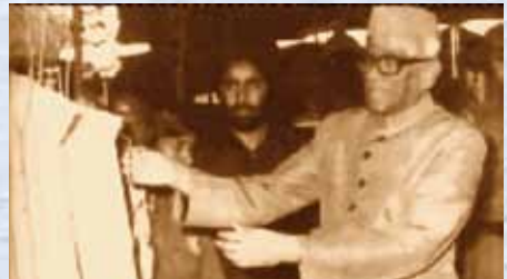
N Sanjeeva Reddy, laying foundation stone for Headquarters Building
