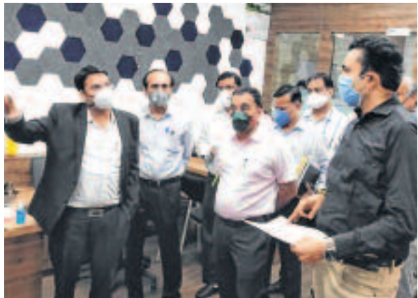
Energy secretary Akash Tripathi inspecting smart meter control room at West Discom office on Saturday.
